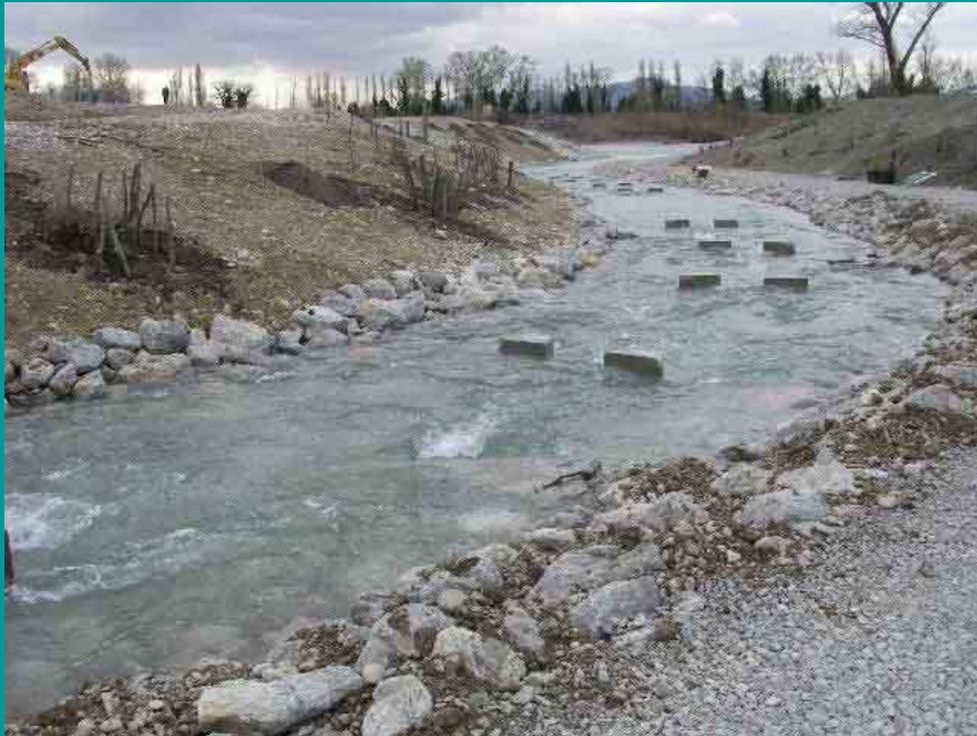
Artificial bypass chanel La Drôme
