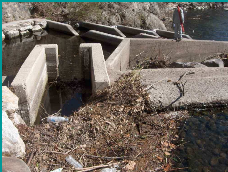
Lack of maintenance (BSN dam, Ardèche)
